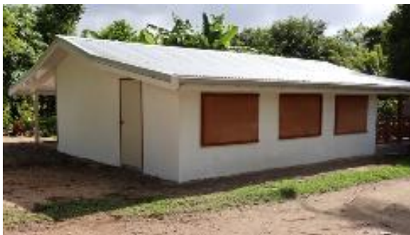
Figure 4 Accessible Ablution block for Sola market house, Vanualava
