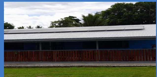
Image 3: Solar panels installed on the roof of the Penama Skills Centre
