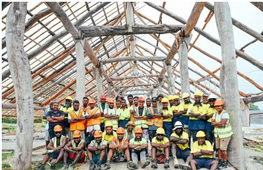
Image 4: Trainees working on the construction of the Chiefs' Nakamal in Port Vila.
