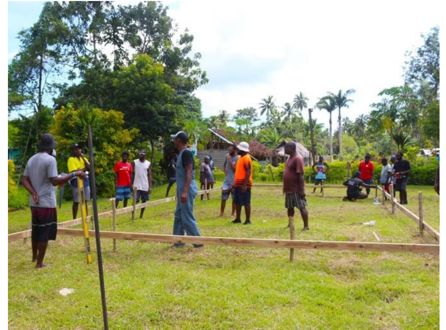
Image 9: Plumbing graduates applying new skills with the construction of WASH infrastructure in Santo
