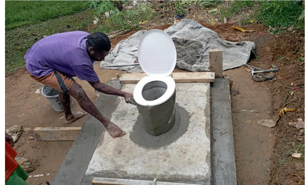
Image 5: West coast Santo plumber installing VIP toilet*
