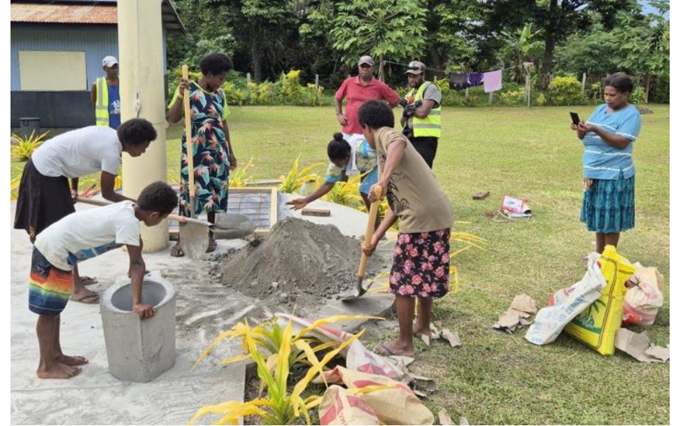
Image 3: VIP toilet slab construction involving women and youth in South Ambae
