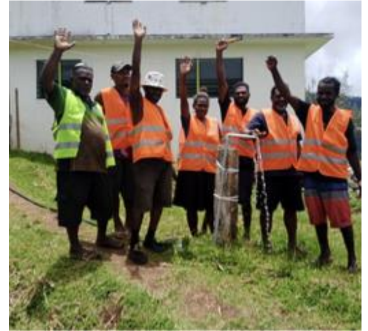
Image 8: Plumbing trainees and the assistant trainer standing behind a tap stand they installed as part of the practical training for Certificate II in Plumbing delivered at Melsisi
