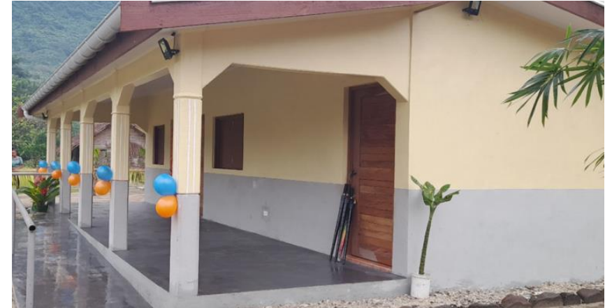
Image 7: Opening of the Ureparapara Fish Market, with accessible ramp, in Divers Bay, Torba, in April
