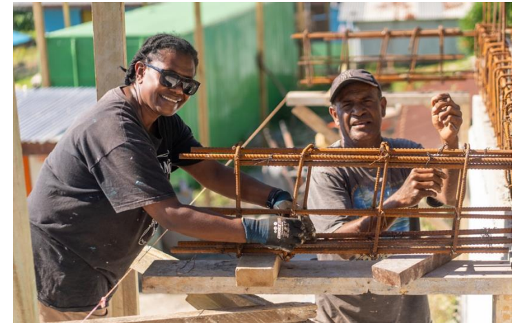
Image 5: Serel and her husband, Guytou at work together on site.
