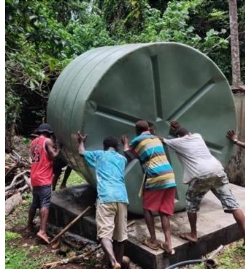
Image 11: Tavolavola community members in North Ambae helping to move a water tank into position.
