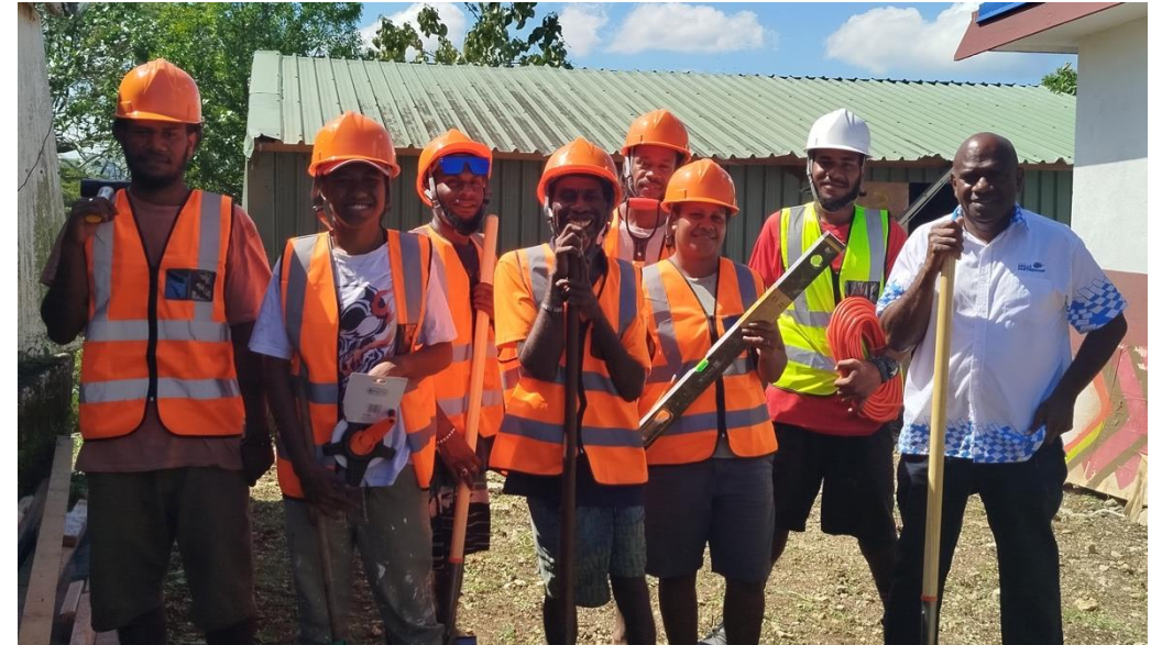
Image 2: SATOMAFEA construction workers onsite, to begin their first contract to build the accessible washroom facility at the National Chief's Nakamal, Port Vila.
