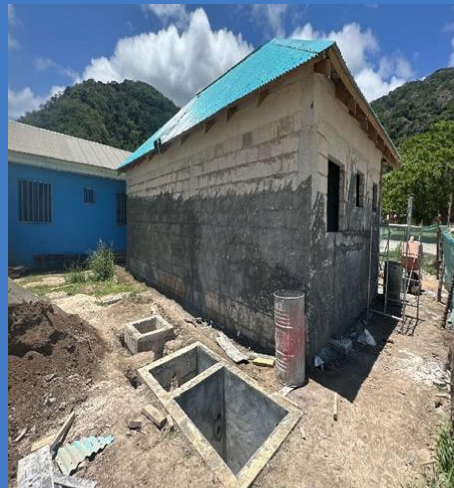
Image 5 : Completion of septic works as part of construction
