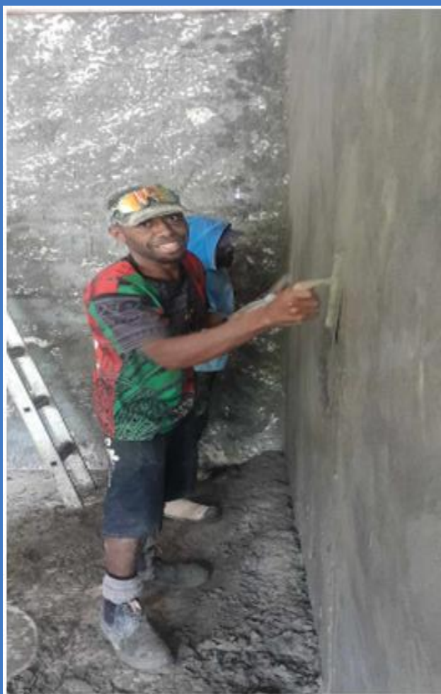
Image 4 : Mr. James Manai from MNCS Construction Company undertaking the plastering works
