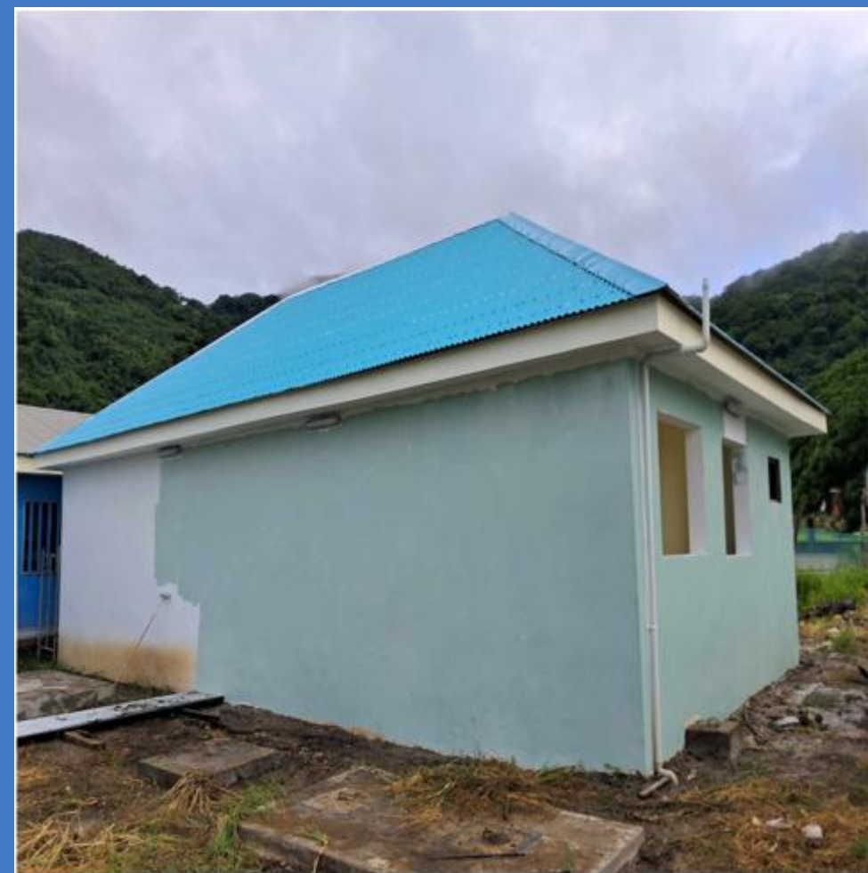
Image 3: Painting works being completed on the VTIC building
